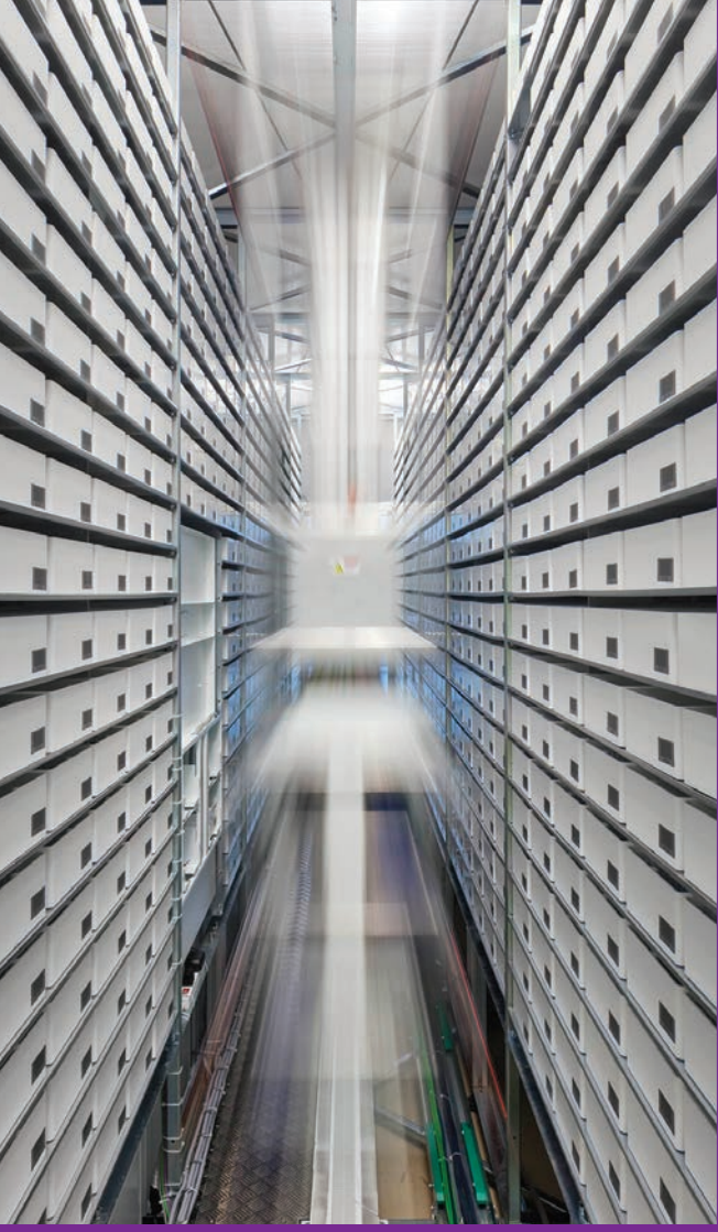
Humber River Hospital's digital pill-picker at work.
